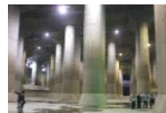
The metropolitan area outer underground discharge channel
